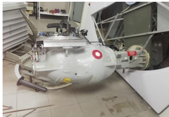
Figure 4. Dismantling process of collimator head
